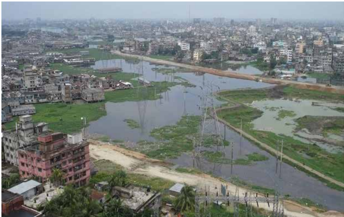
Overview of the Lake prior to the project © Vitti Sthapati Brindo Limited
