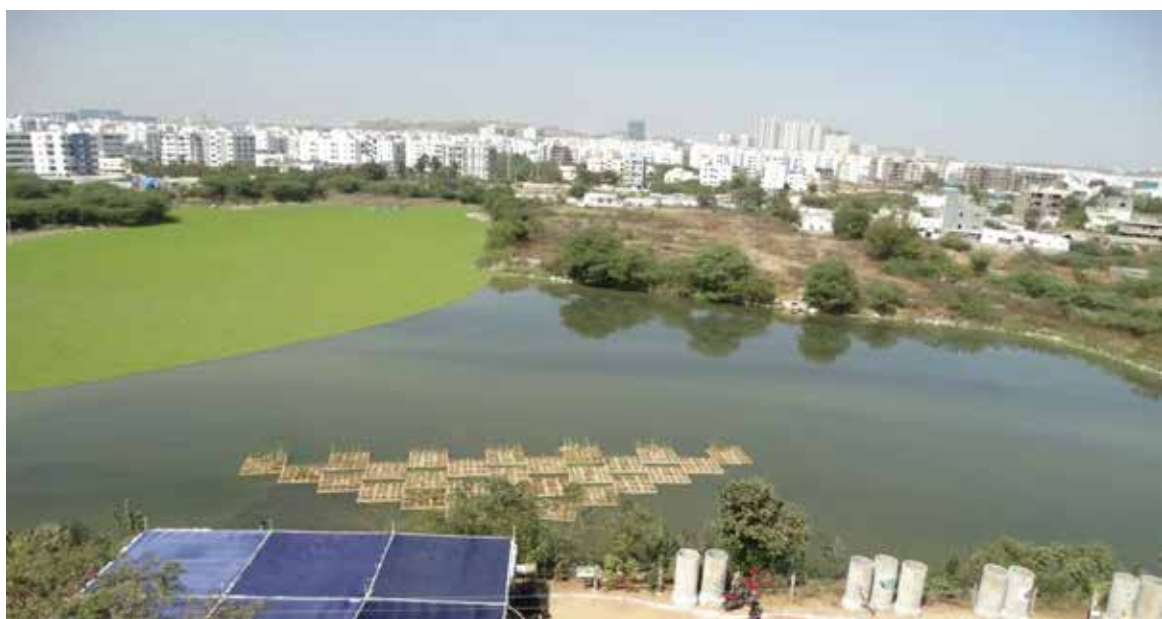
Floating treatment wetland technique being applied in the lake © Madhulika Sharma Choudhary
